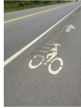
Shoulder Bike Lane with Rumble Strip Source: Corey Hull, SGRC
