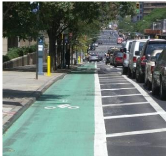
Protected bike lane in New York City Source: Jim.henderson- Wikimedia Commons 25
